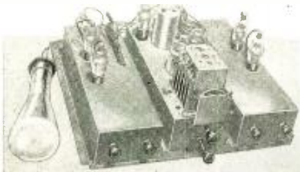
Fig. 3—The interior of the Emyradio television receiver—small model.
